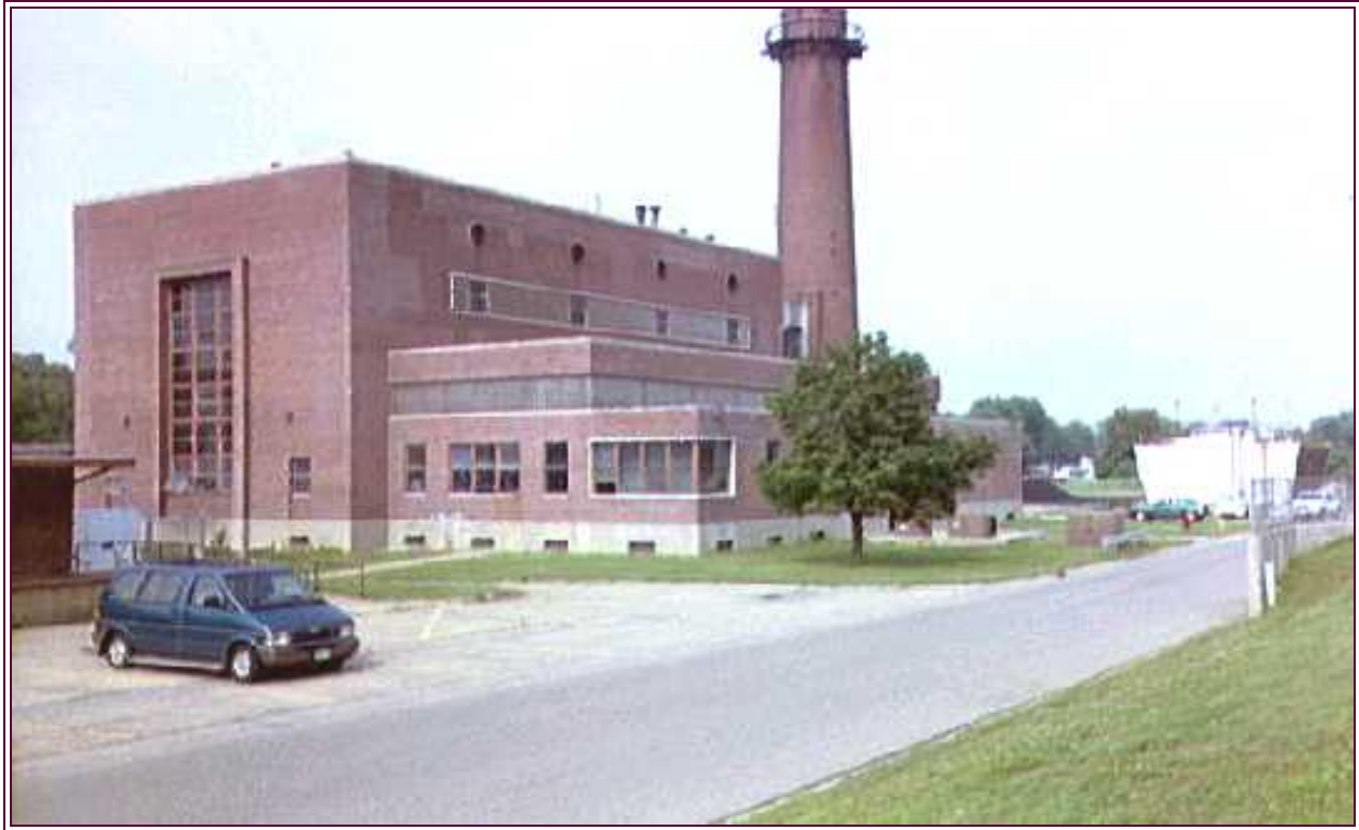
Figure 3. Lincoln Development Center Boiler House
