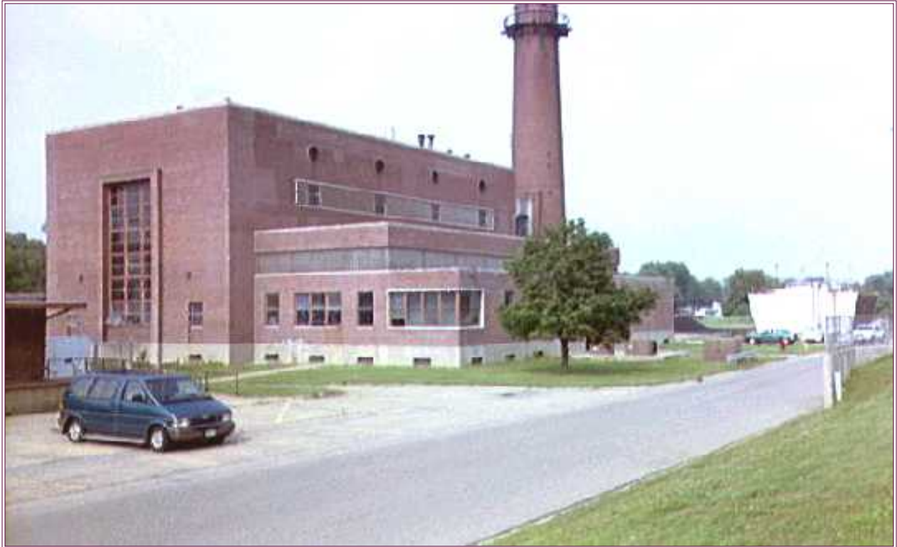
Figure 3. Lincoln Development Center Boiler House
