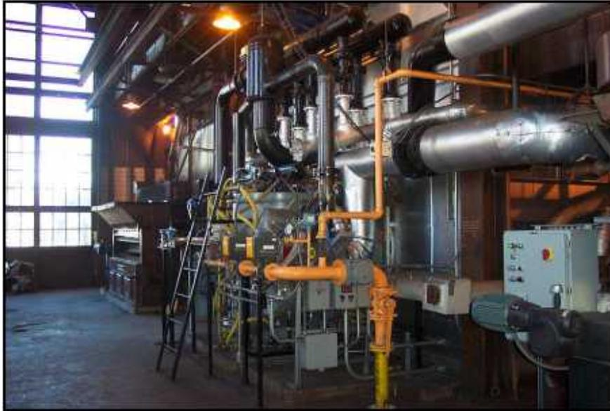
Figure 7. Ashworth 40 x 10<sup>6</sup> Btu/hr 3-Stage Combustion System.
