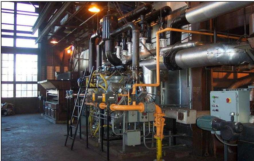
Figure 6. Ashworth  $40 \times 10^6$  Btu/hr 3-Stage Combustion System.
