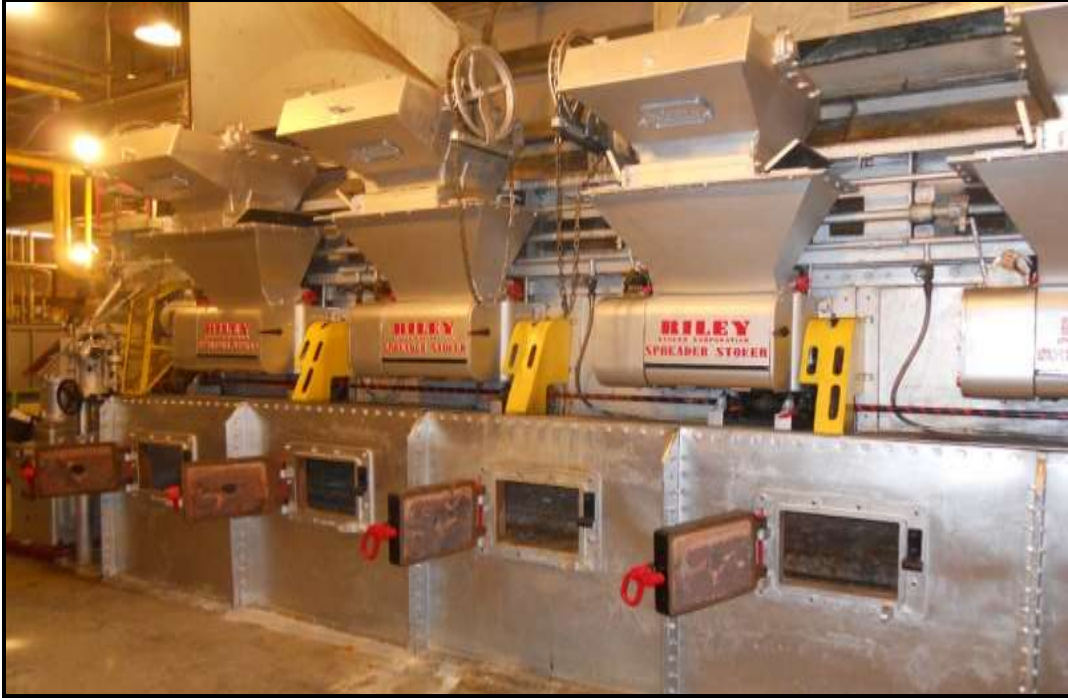
Figure 6. Unit #5 - Travelling grate stoker.
