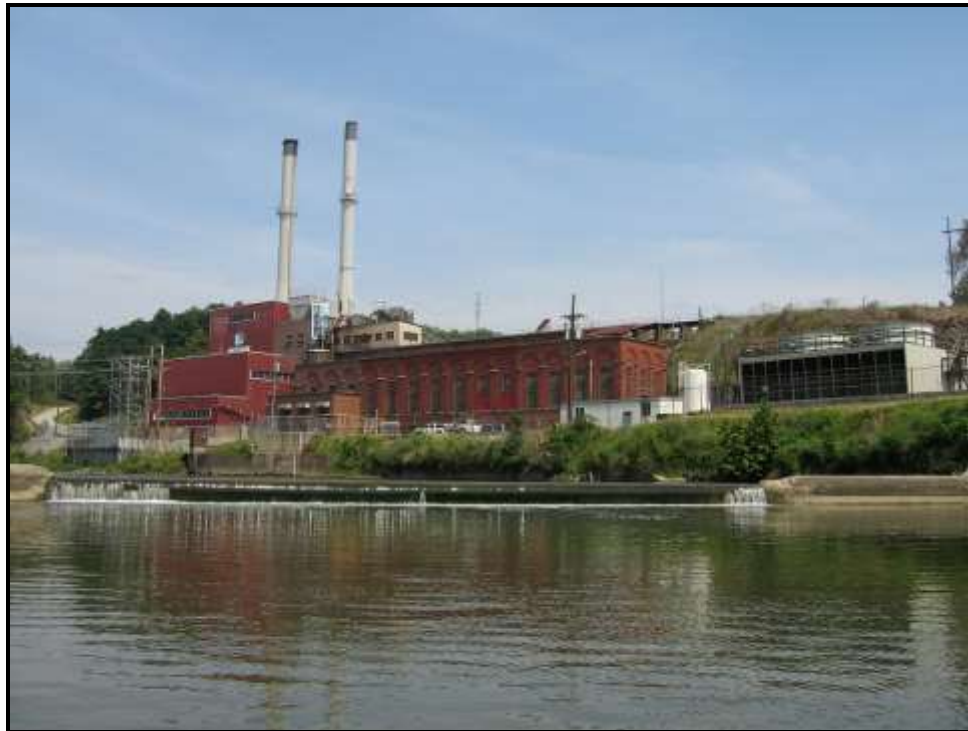
Figure 1. Crawfordsville Power Plant.
