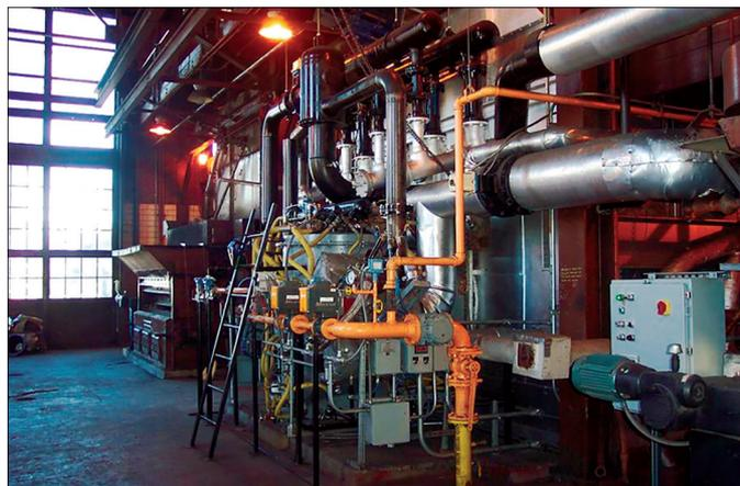
**FIGURE 2. Ashworth Gasifier-Combustion system (40 million Btu/hr)**
